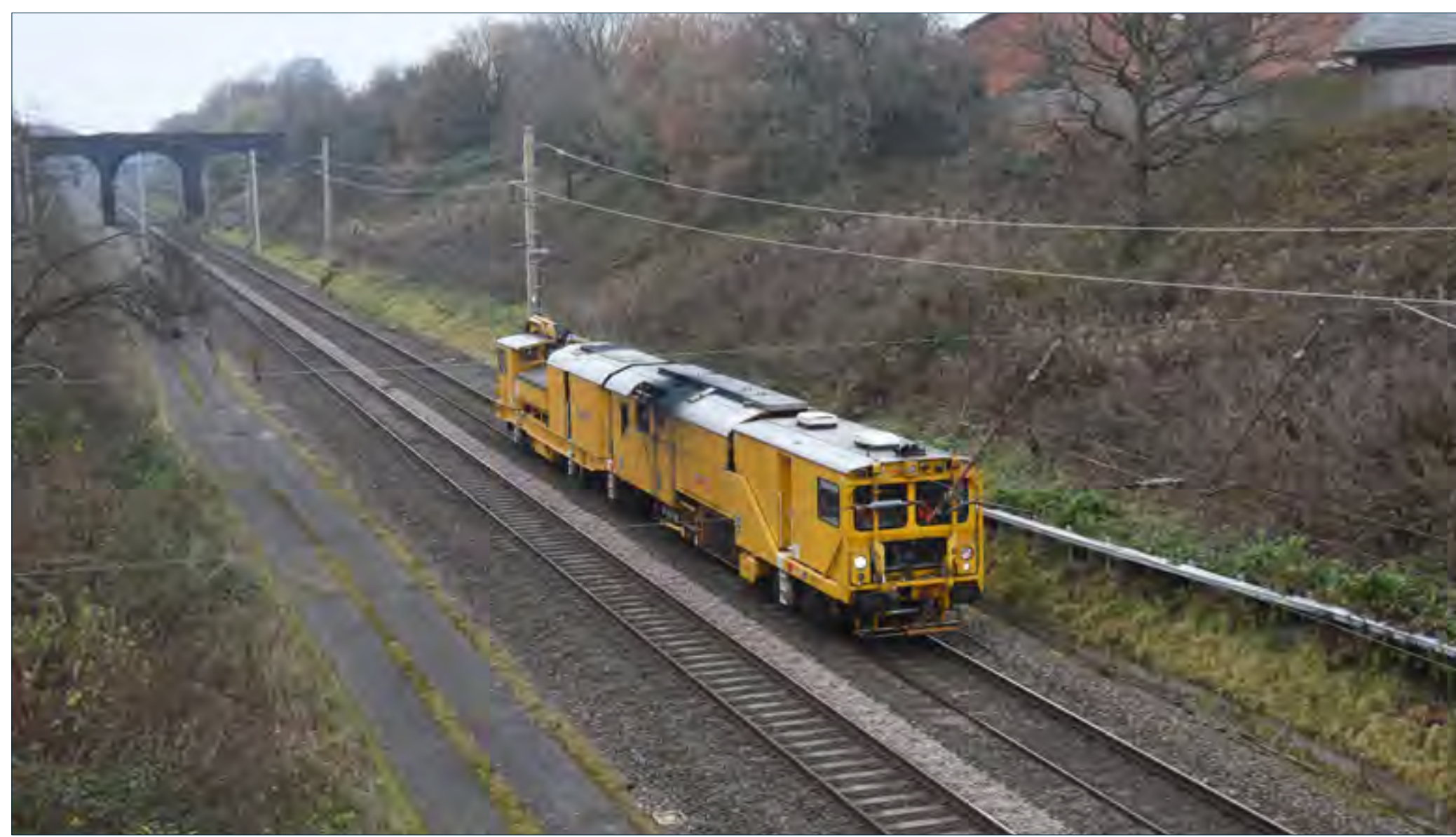
◀ A Network Rail Stoneblower heads along the West Coast main line at Charnock Richard on November 23rd. John Sloane
