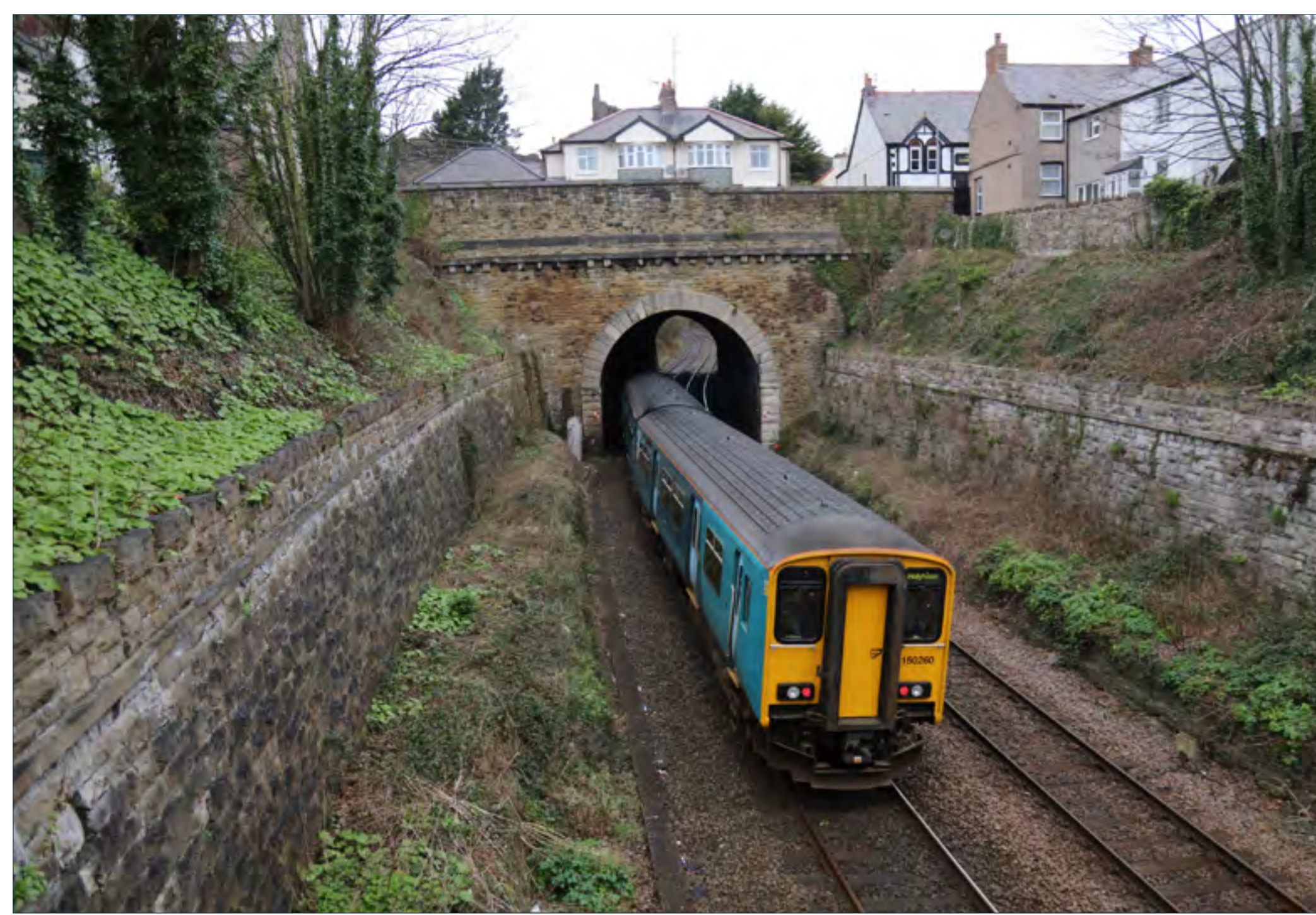
▶ 'The Railroad Runs Through the Middle of the House' was a popular song when I was a young lad...and here Class 150 260 passes beneath a pair of semi-detached houses in Upper Gate Street as it departs Conwy on February 19th with the 07:21 Cardiff - Holyhead service. Jeff Nicholls
