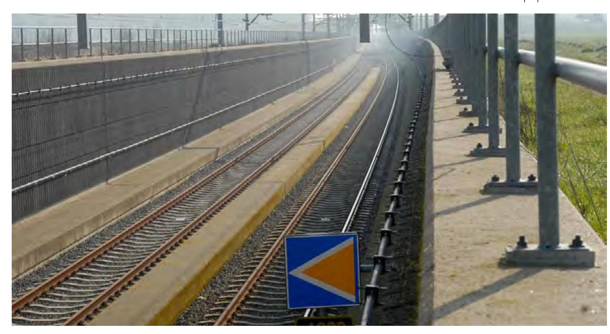
Alstom's Atlas ERTMS Level 2 is a digital signalling solution that allows trains to run at higher speeds without physical lineside signals. With Atlas, the Valladolid-León line will see an increase in safety and availability, as well as in train speed, with maximum speeds increasing from 200 km/h to 300 km/h. The resulting updated timetable will allow passengers to benefit from shorter journey times.
