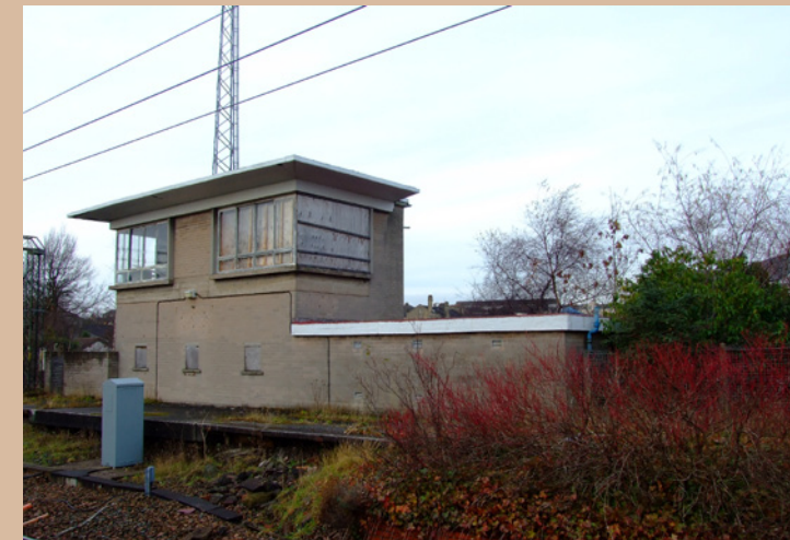
A general view of the old and disused Airdrie station signal box which is due to be demolished next year and replaced with a brand new platform and the foilage below, replaced with new track as part of the Airdrie - Bathgate (A - B) Project.
