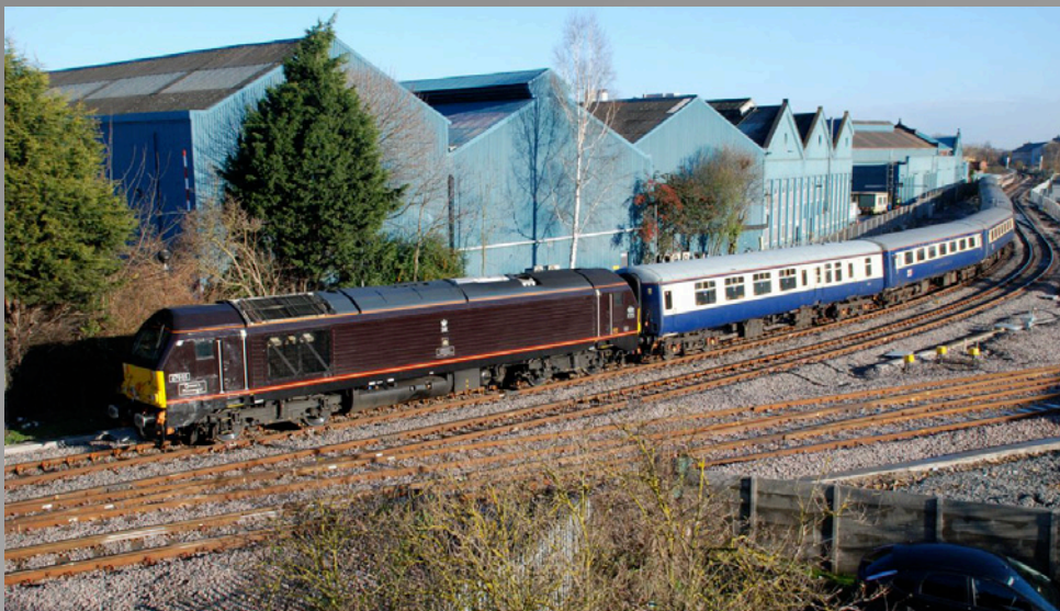
Below: Class 67 005 on the rear of 5227 negotiates the realigned Pelham Street Junction, Lincoln, en route to Barnetby, where the train was stabled and made ready for the return. Steve Thompson
