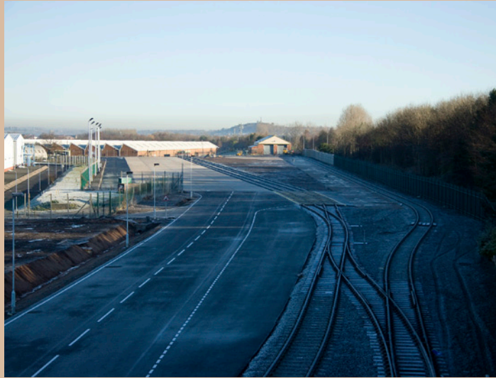
Above: Looking East with Lilleshall hill in the distance. The old MOD 2 road engine shed is also visible. These are the new loading sidings.
