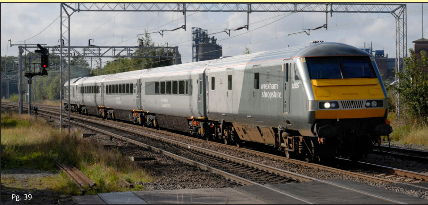
Left: The first rake of refurbished Mk III stock for the Wrexham, Shropshire and Marylebone Railway was delivered at the beginning of September and was tested in a series of circular proving runs from Crewe. On the morning of Wednesday 9th September, the 5Z01 Crewe - Shrewsbury - Crewe trial train comprising DVT 82305, buffet/first 10218, standard open 12145 and standard open 12127, propelled by locomotive Class 67 010, all in the WSMR livery, moves away from Bushbury Junction, Wolverhampton, West Midlands.
