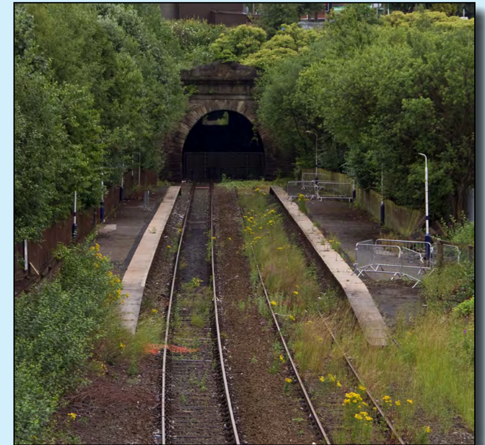
Another view of Werneth showing gated tunnel and disused station
