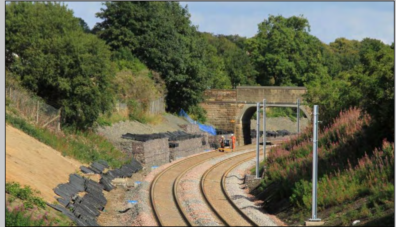
Above: With the trackwork almost complete the embankments get tidied up and drainage installed. Jonathan McGurk Below: The stations are in place for the electrification team to start the task of wiring the route. Jonathan McGurk
