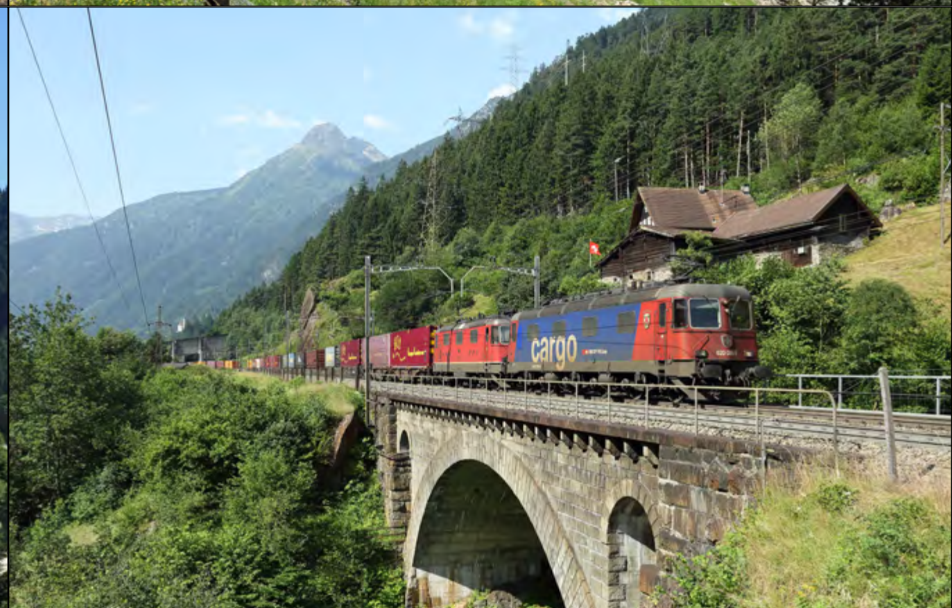
SBB Cargo Class 620.086 and Re 4/4 ii No. 11345 approach Gurnellen whilst hauling intermodal train No. 40126 Chiasso - Basel. Laurence Sly
