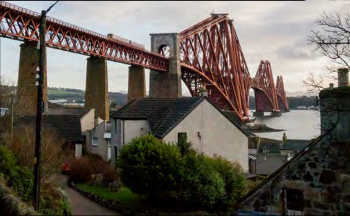
On February 3rd, a Scotrail Class 158 is seen crossing the Forth Bridge whilst working the 2K05 14:40 Edinburgh Waverley - Glenrothes with Thornton via Kirkcaldy service. Jonathan McGurk
