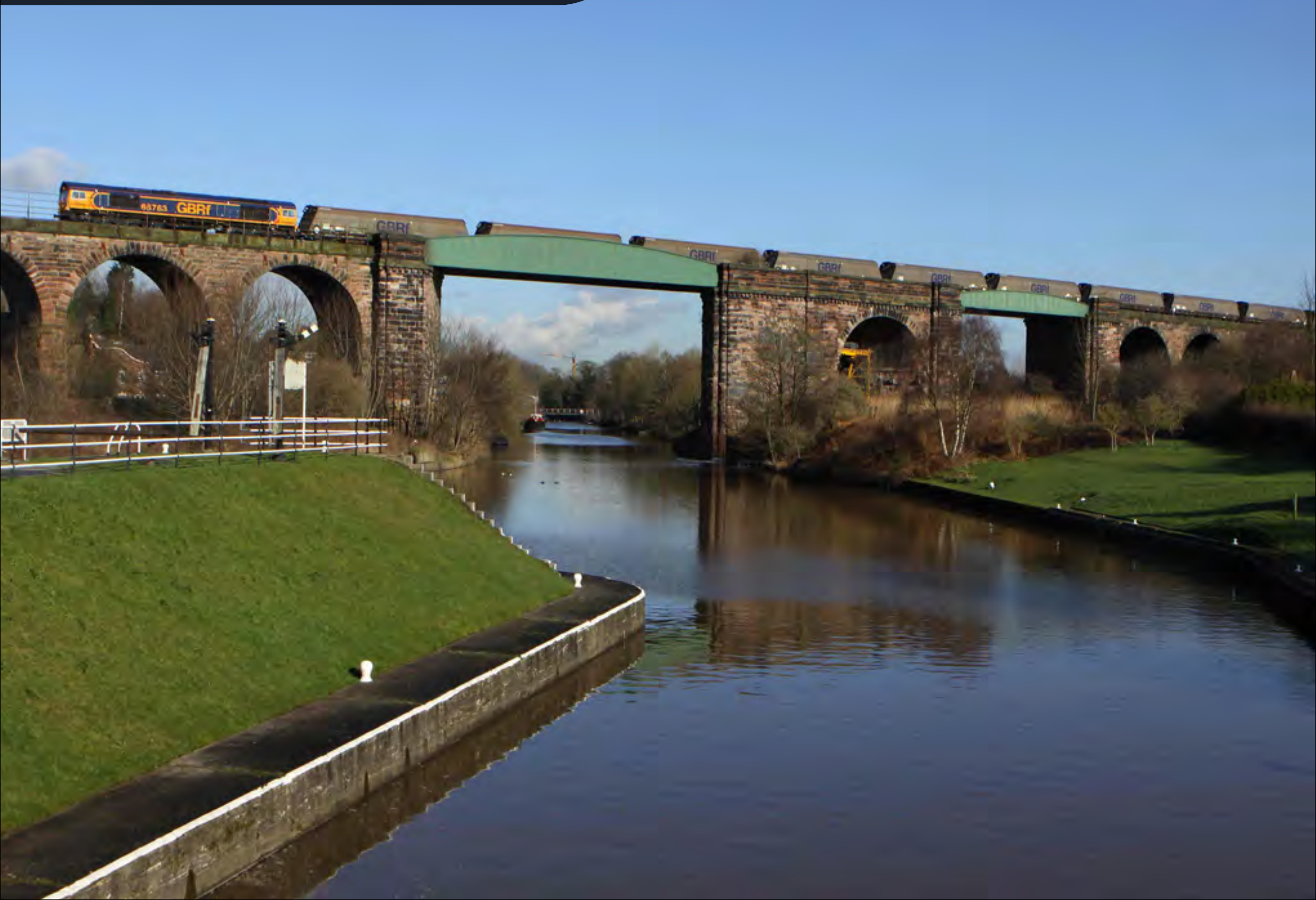
On February 23rd, Class 66 763 is photographed crossing Northwich Viaduct, heading over the River Weaver at Hunts Lock working the 4M12 06:00 Drax - Liverpool Bulk Terminal empty Biomass. Nick Clemson
