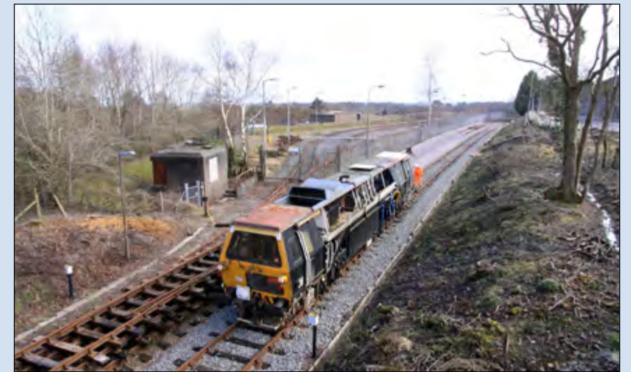
Furzebrook to Creech Bottom track tamping on March 5th.
