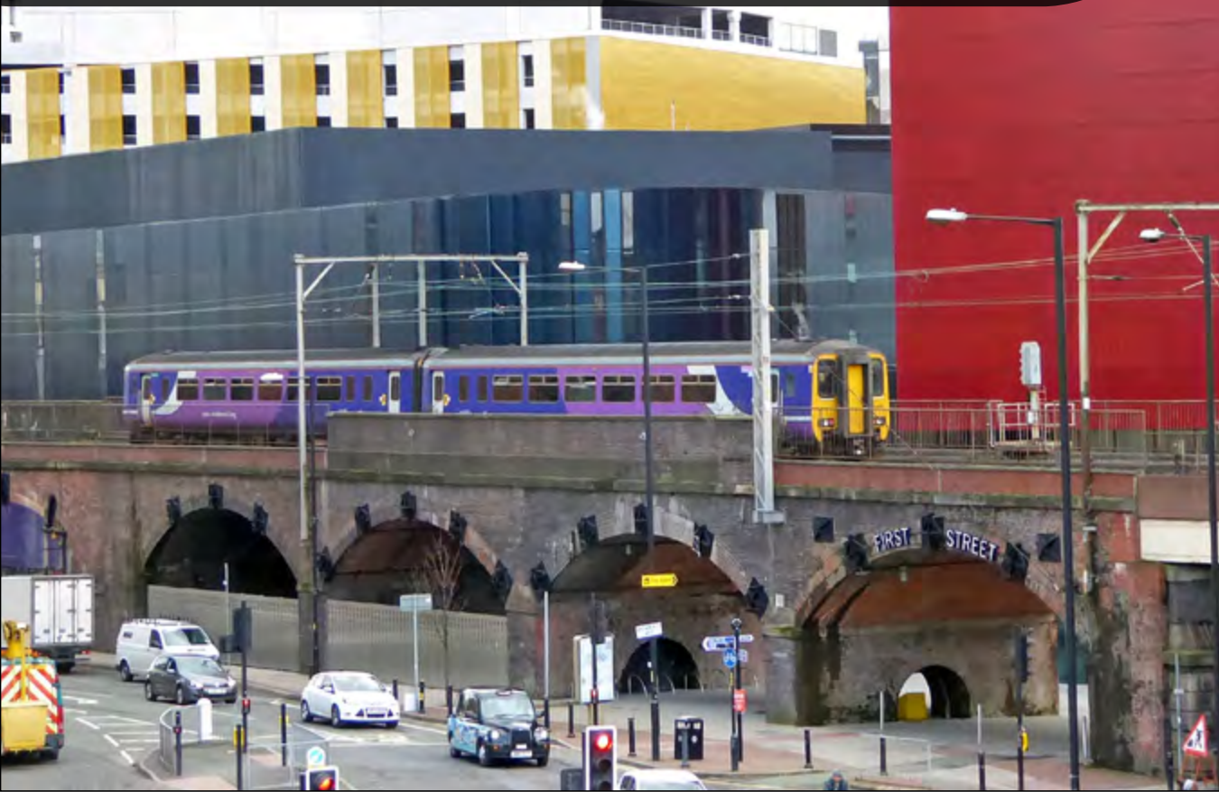
On March 3rd, an unidentified Northern Rail Class 156 DMU passes over the arches between Deansgate and Manchester Oxford Road. Michael Lynam
