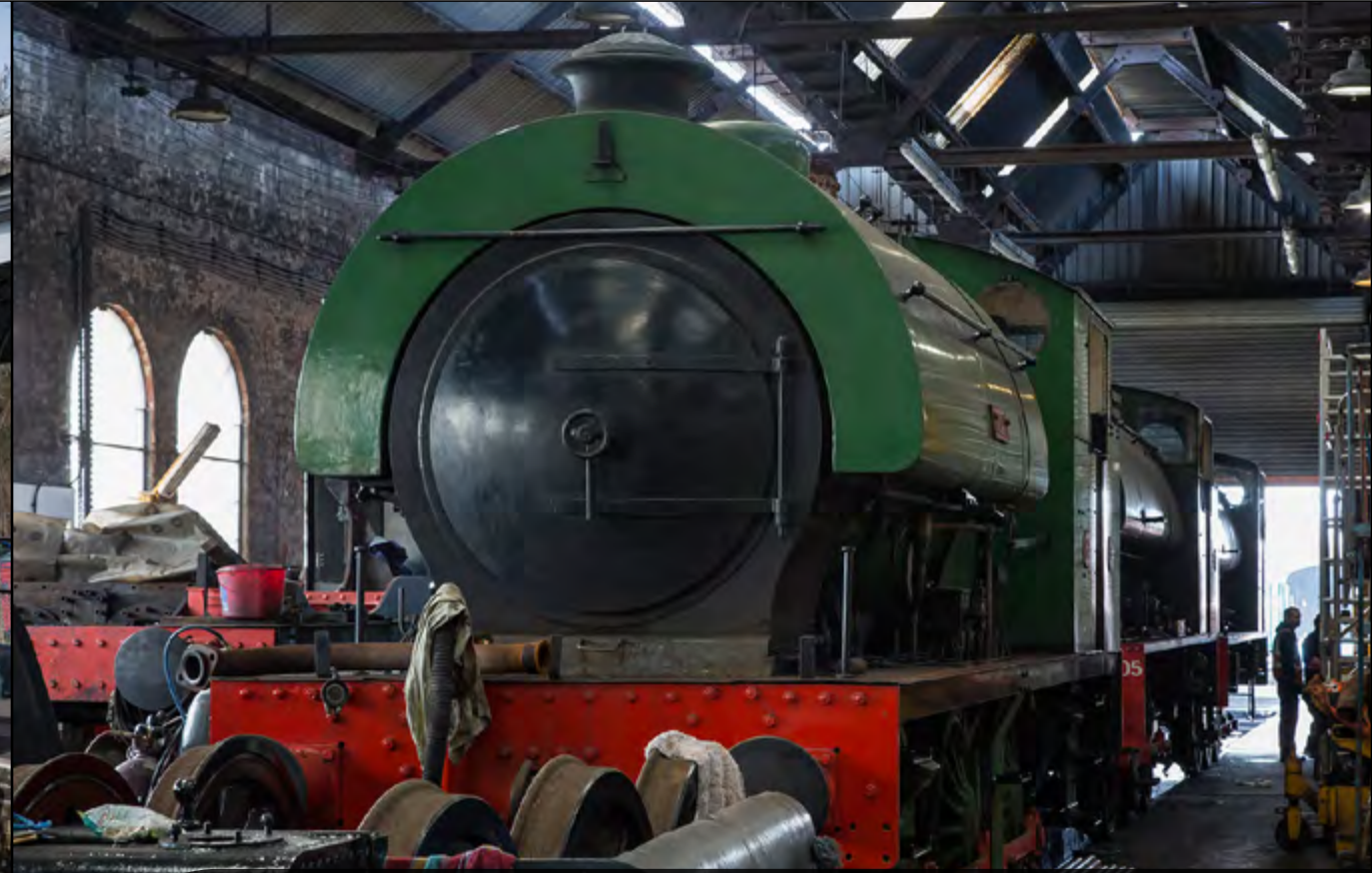
RSH No. 62 'Ugly' is seen under repair in the shed at Tunbridge Wells West on April 2nd. Richard Hargreaves
