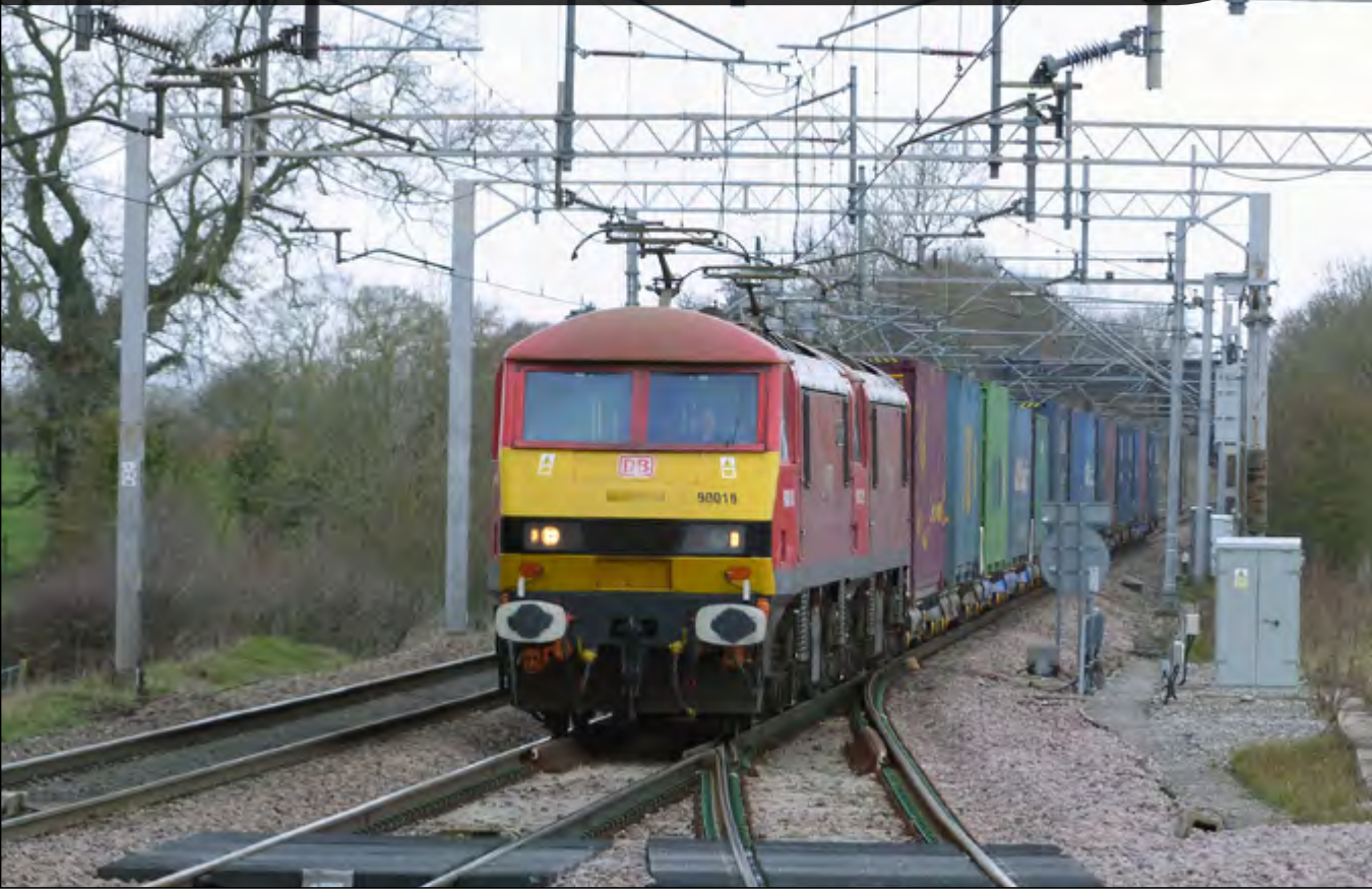
Class 90 018 and 90 029 head a Mossend - Daventry intermodal through Acton Bridge on April 7th. Michael Lynam
