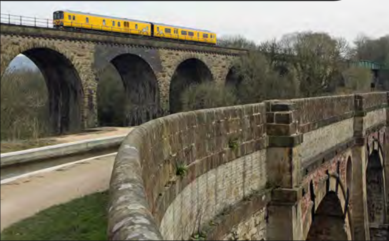
Class 950 001 crosses Marple Viaduct on April 11th with the 06:41 Derby RTC - Longsight. Marple Aqueduct carries the Peak Forest Canal 100 feet above the River Goyt. Nick Clemson
