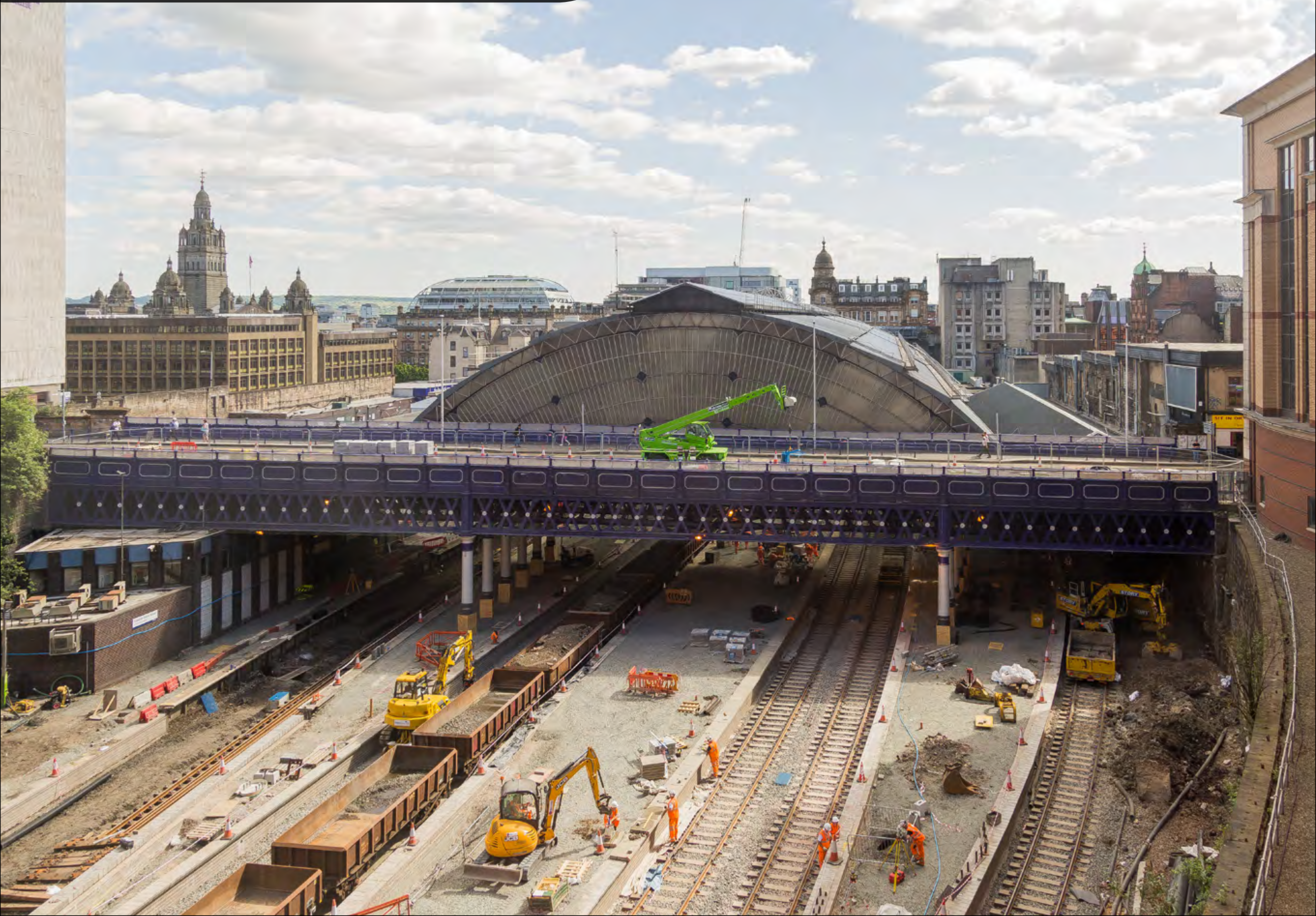
A look at the E.G.I.P. Project Works taking place at Glasgow Queen Street station on June 2nd. Jonathan McGurk
