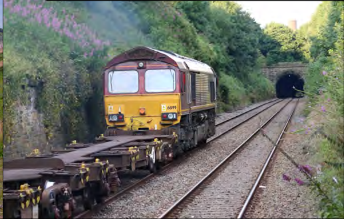
Class 66 199 heads towards Upholland tunnel on July 19th working the 6E16 Knowsley Freight Terminal - Wilton EFW. Alan Rigby
