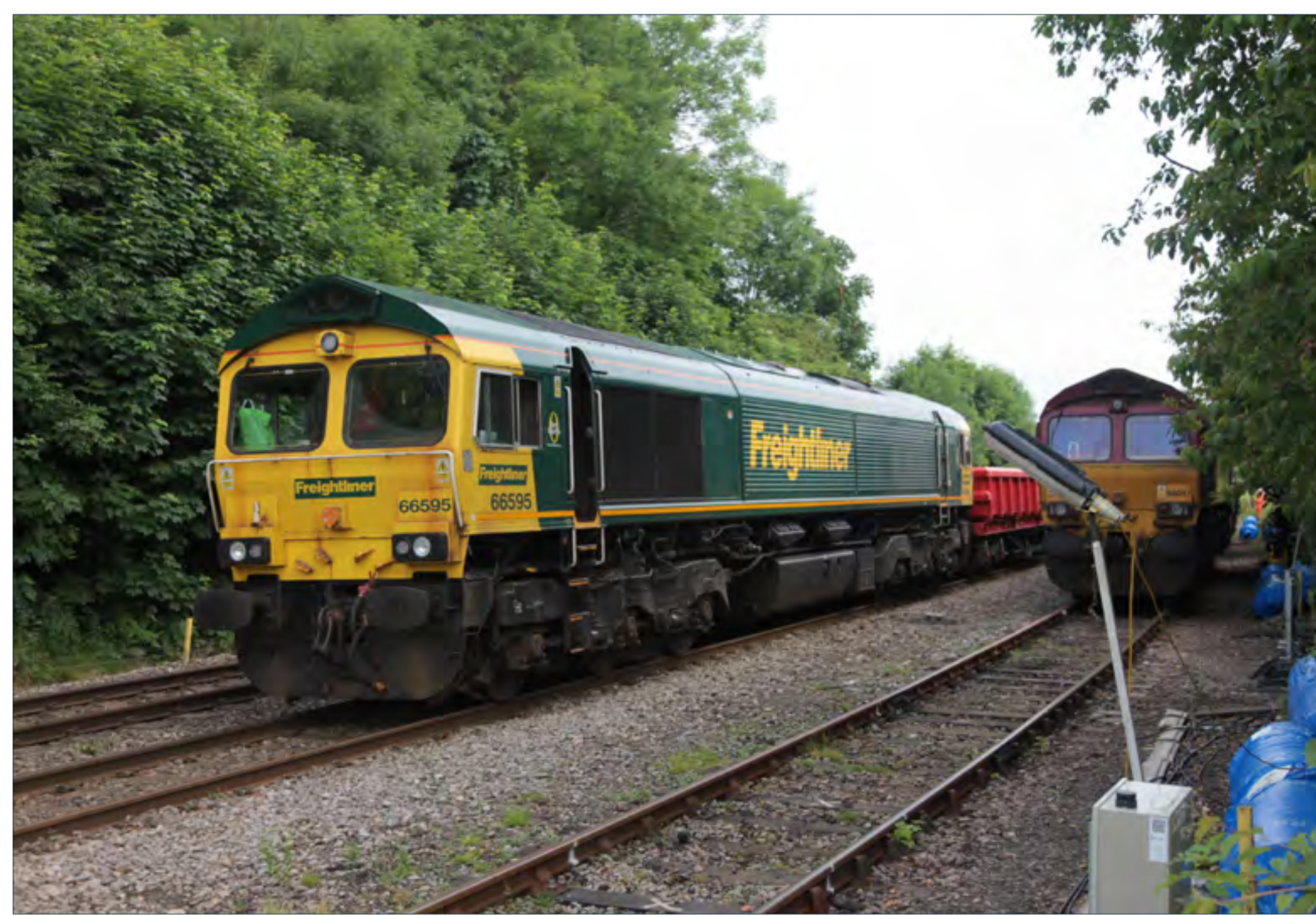
Class 66 595 and 66 047 are pictured at Malvern Wells during track re-laying works. Neil Pugh
