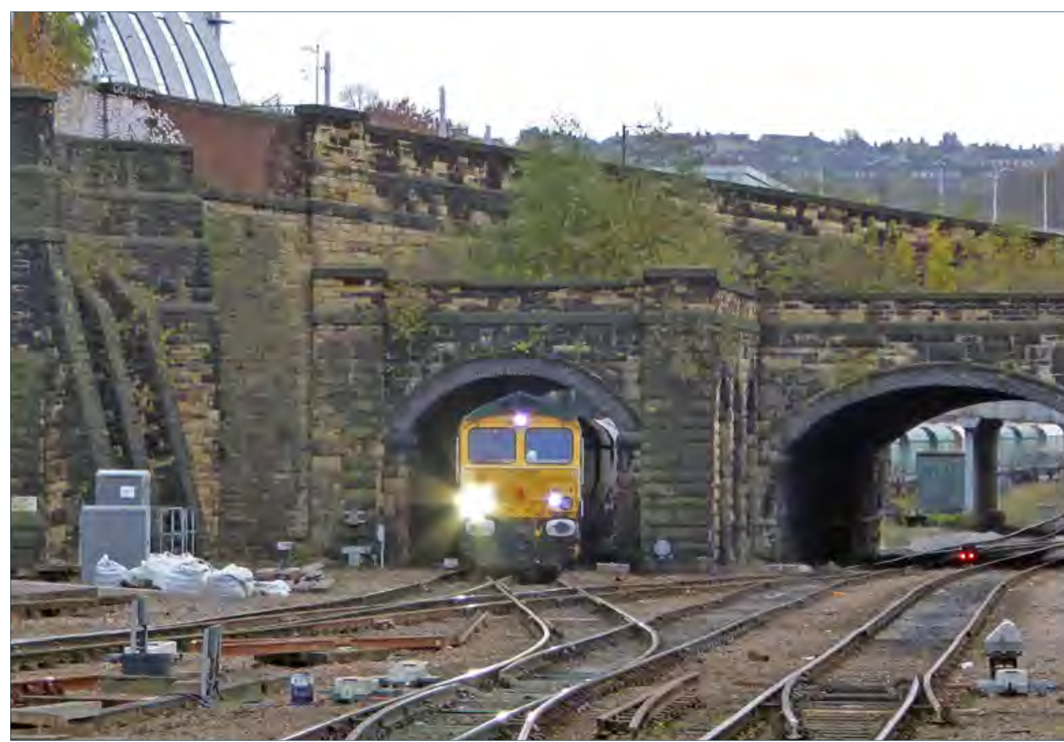
▶ Class 66 614 'Poppy' enters Sheffield station with a stone train from Tunstead Sidings - Brentford Town, November 3rd. Michael Lynam
