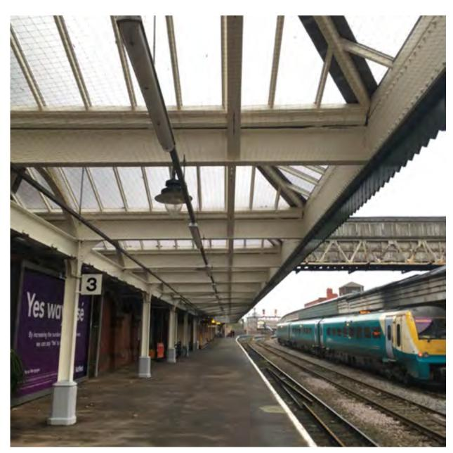
The first phase of work to upgrade Shrewsbury station has been completed as part of Network Rail's Railway Upgrade Plan, to deliver a bigger and better railway for passengers. In July 2016 Network Rail engineers began work to repair and replace the large canopy roof over platforms 3, 4 and 7, which was completed in December.
