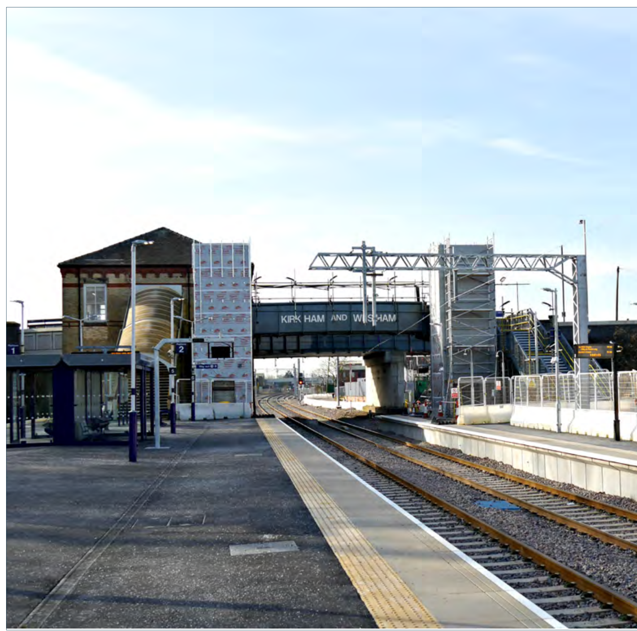
Construction work in progress at Poulton. John Balaam
