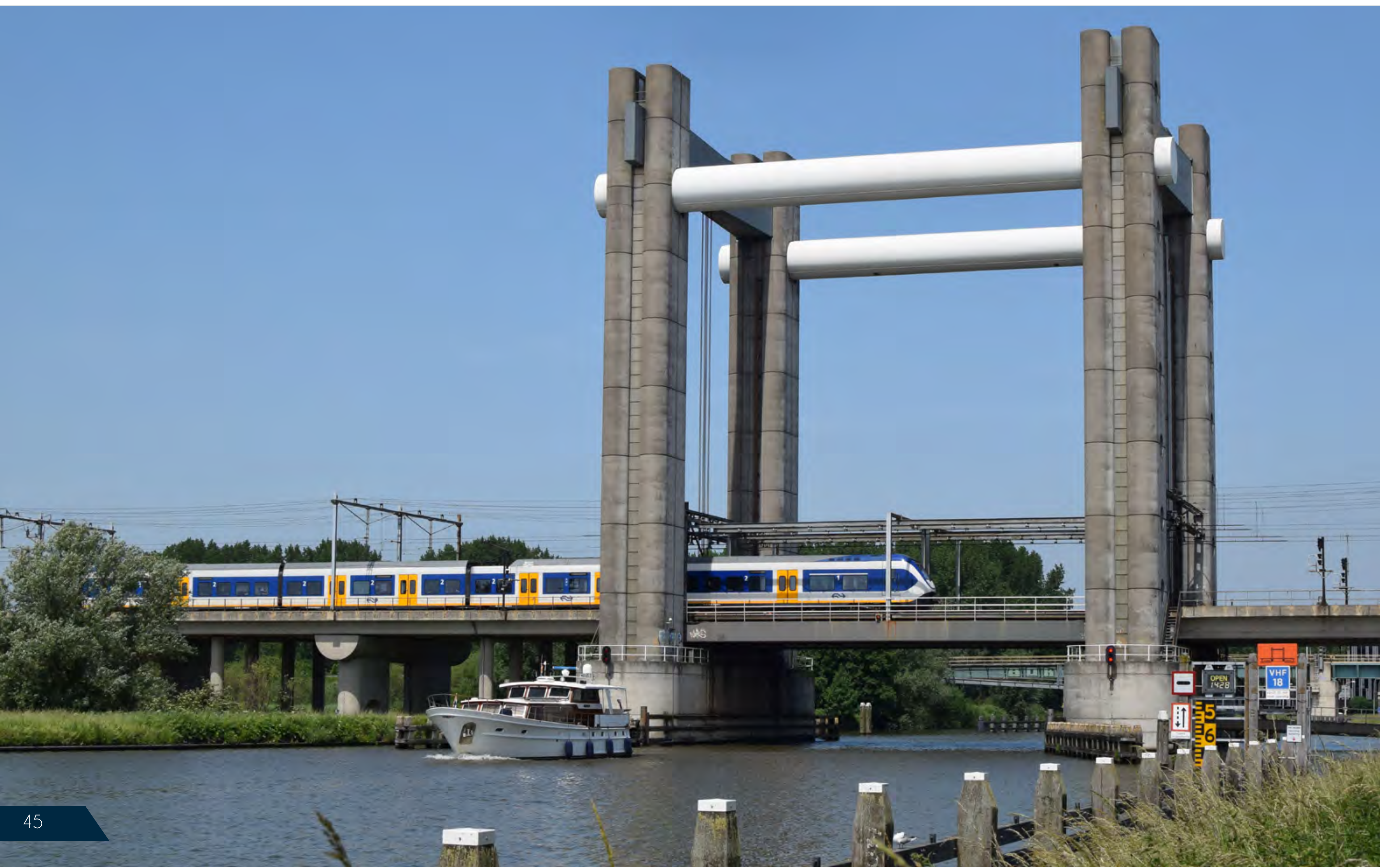
▶ Rail Feeding locomotive BR203 No. 24 runs over the viaduct Stadhouderskade in Rotterdam while the stork takes care of her young ones on May 28th. Erik de Zeeuw
