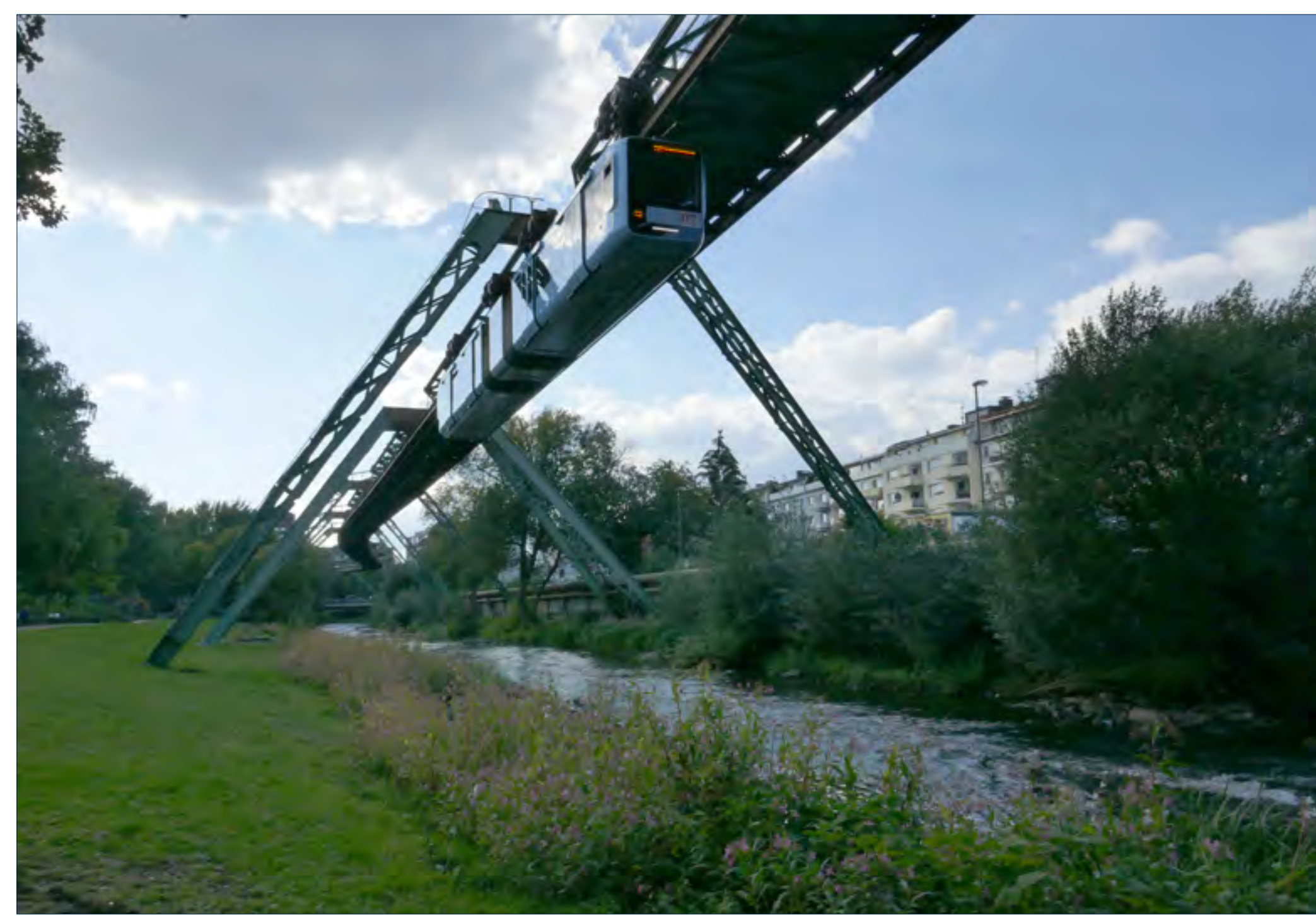
Schwebebahn train No. 02 is seen at Wuppertal Oberbarmen. Stearnsounds
