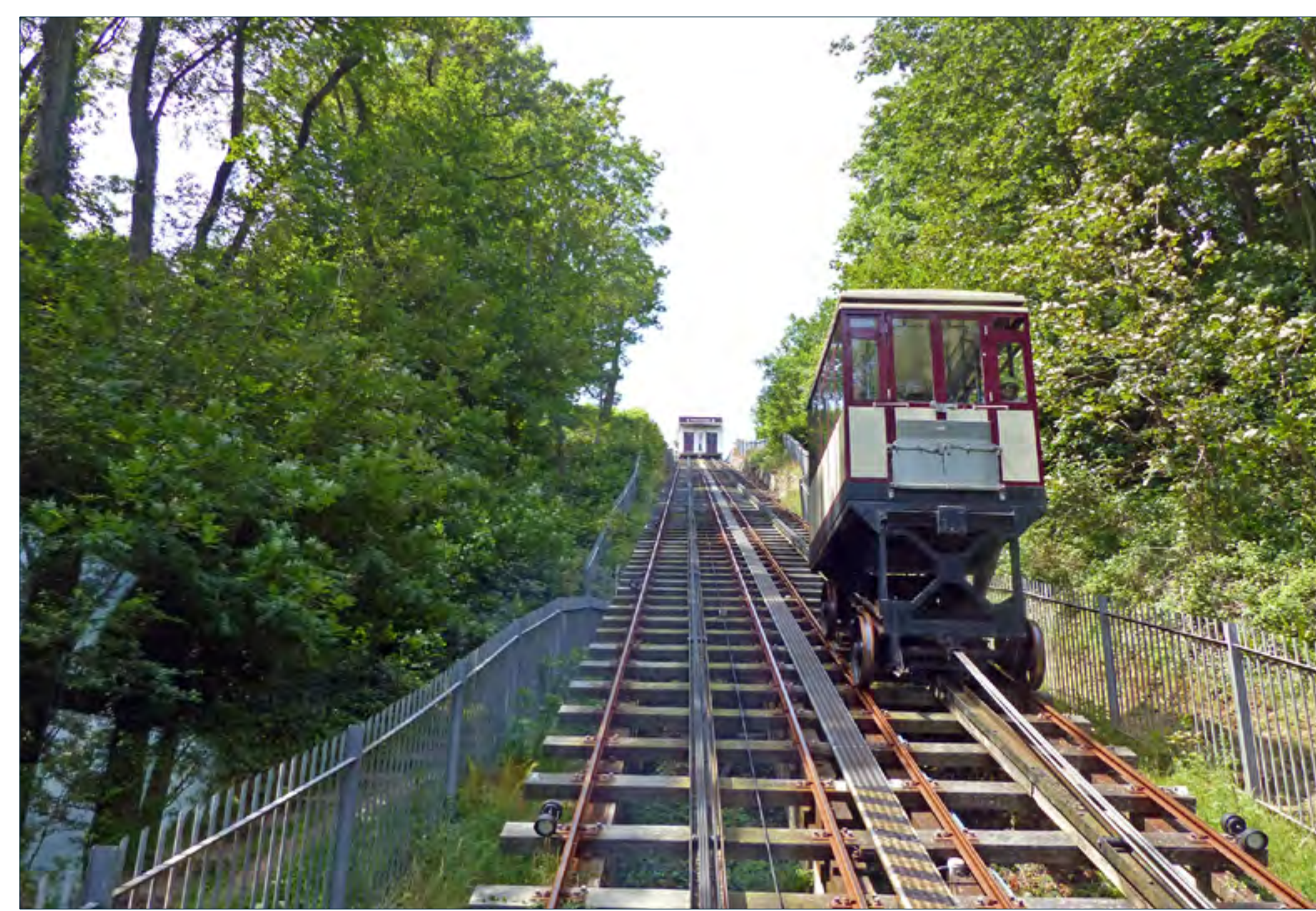
The Babbacombe Cliff Railway was built in 1926 by Waygood Otis, to link Babbacombe (top station) with Oddicombe Beach (bottom beach). Michael Lynam
