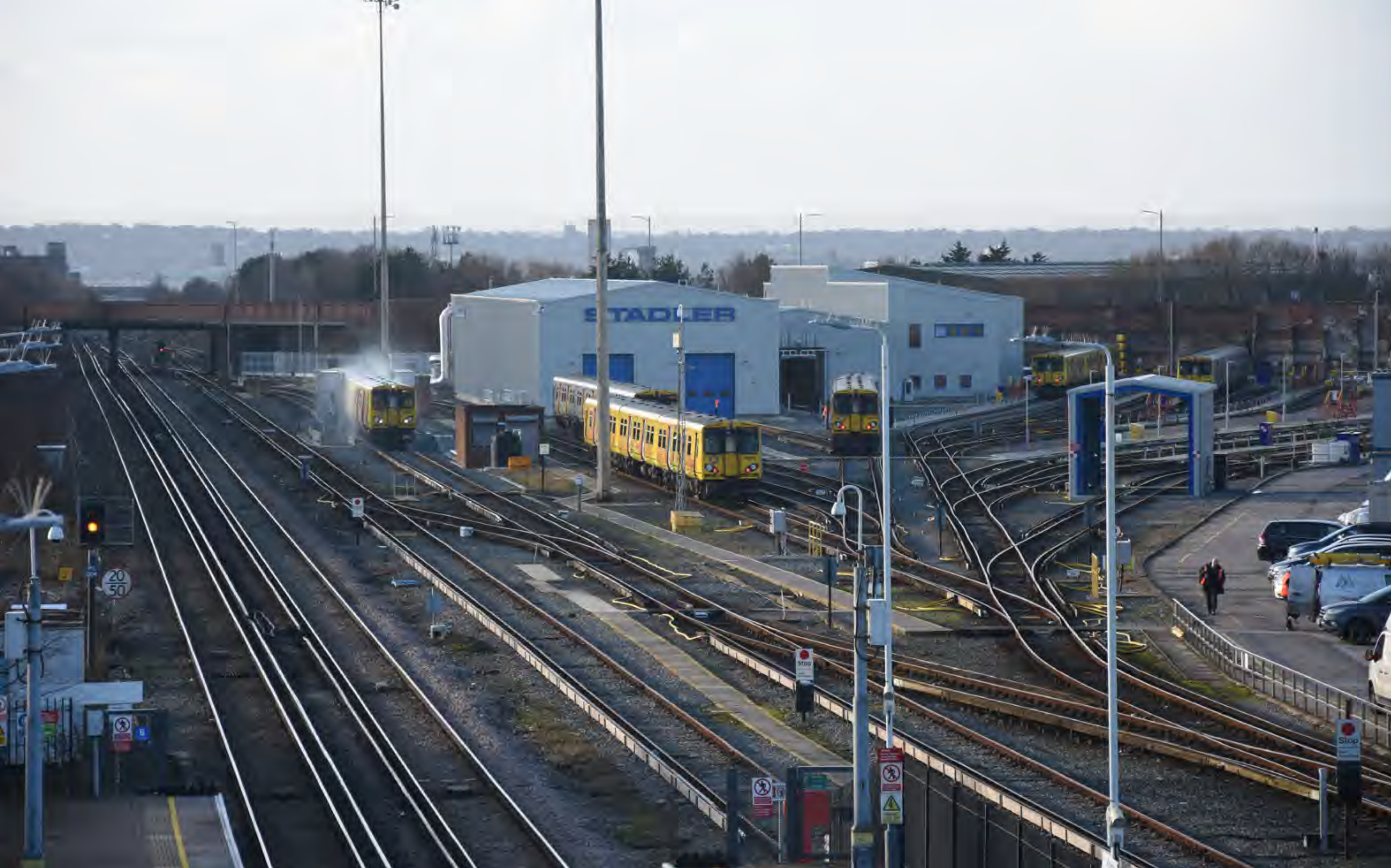
▶ A look at Merseyrail's new Stadler depot at Kirkdale. John Sloane
