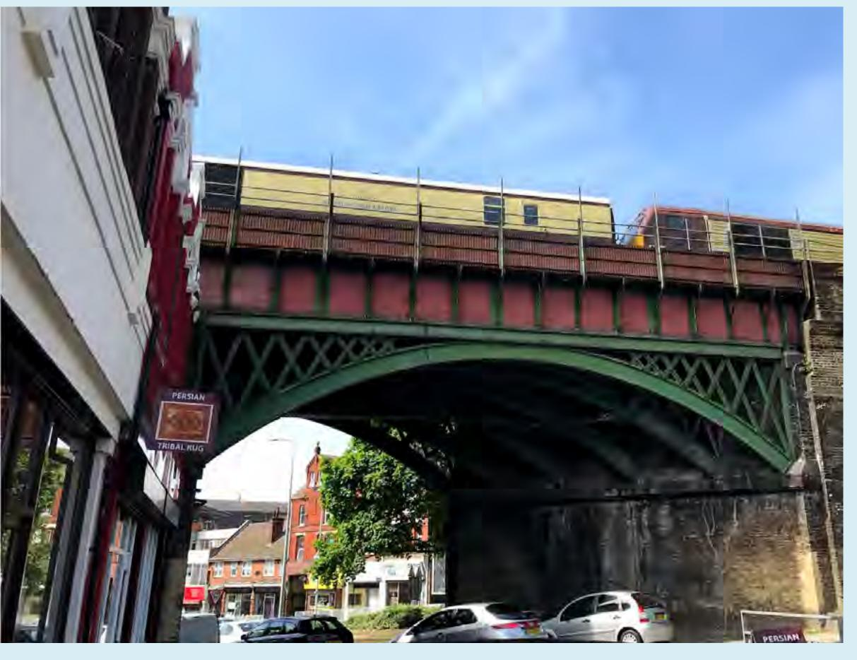
Althoughthestructure is supported by three steel girders, the original cast iron arch girders were left in place for decorative purposes.
