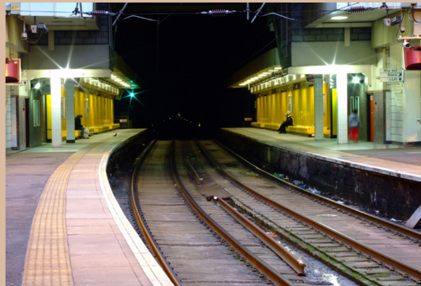
Left: A General View Of Charing Cross Station Looking Towards Glasgow Queen St. Low Level.
