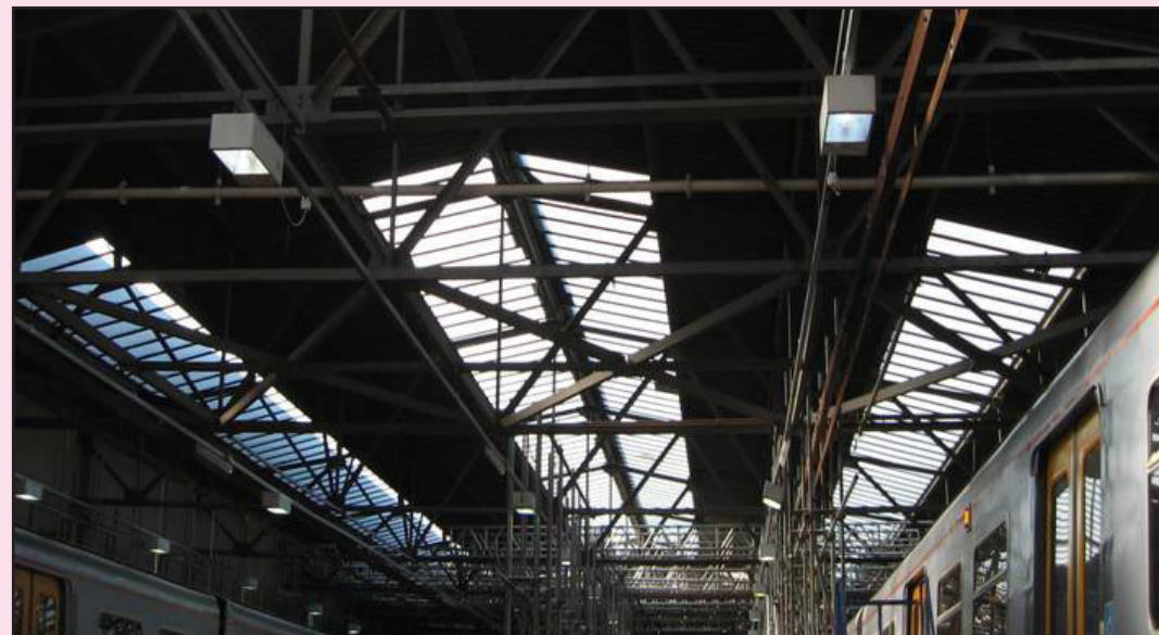
Photo: Inside the depot showing the old roof.
