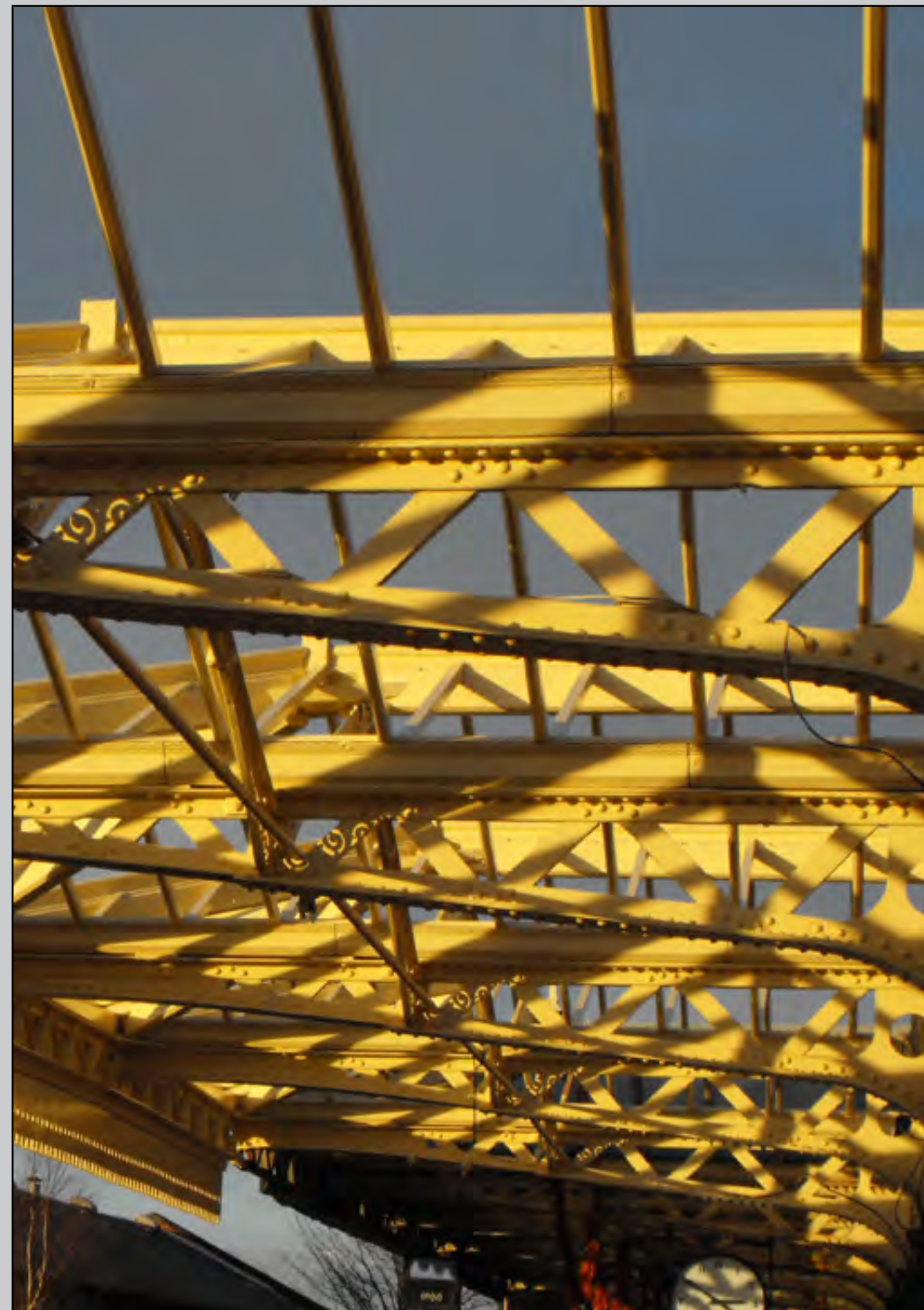
Photo: The sun illuminates the restored canopy on platform 2 in Jan 2012, awaiting the contractors to install the glass. © Tom Ingall
