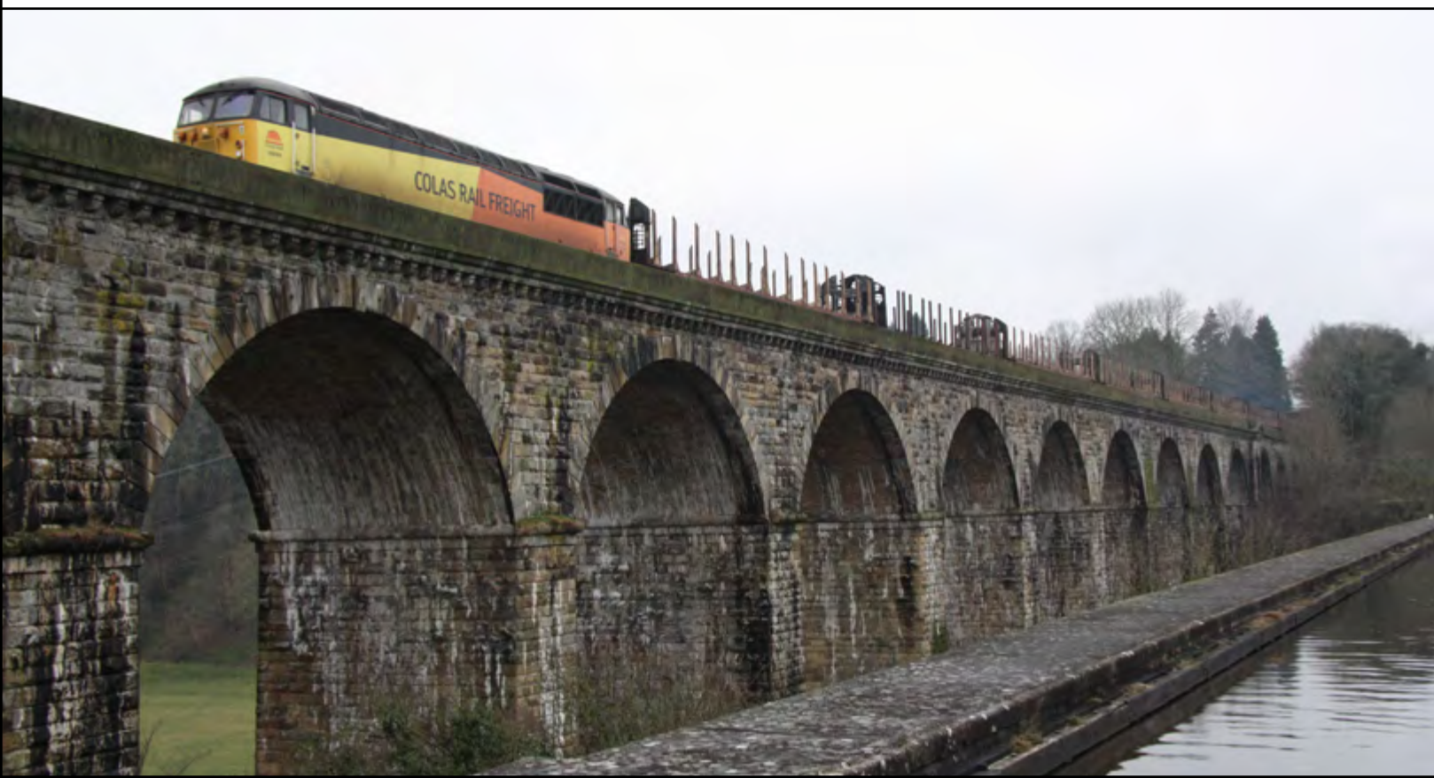
Below: On March 9th, Class 56 094 crosses Chirk viaduct with timber empties from Kronaspan at Chirk heading for Baglan Bay. Phil Martin
