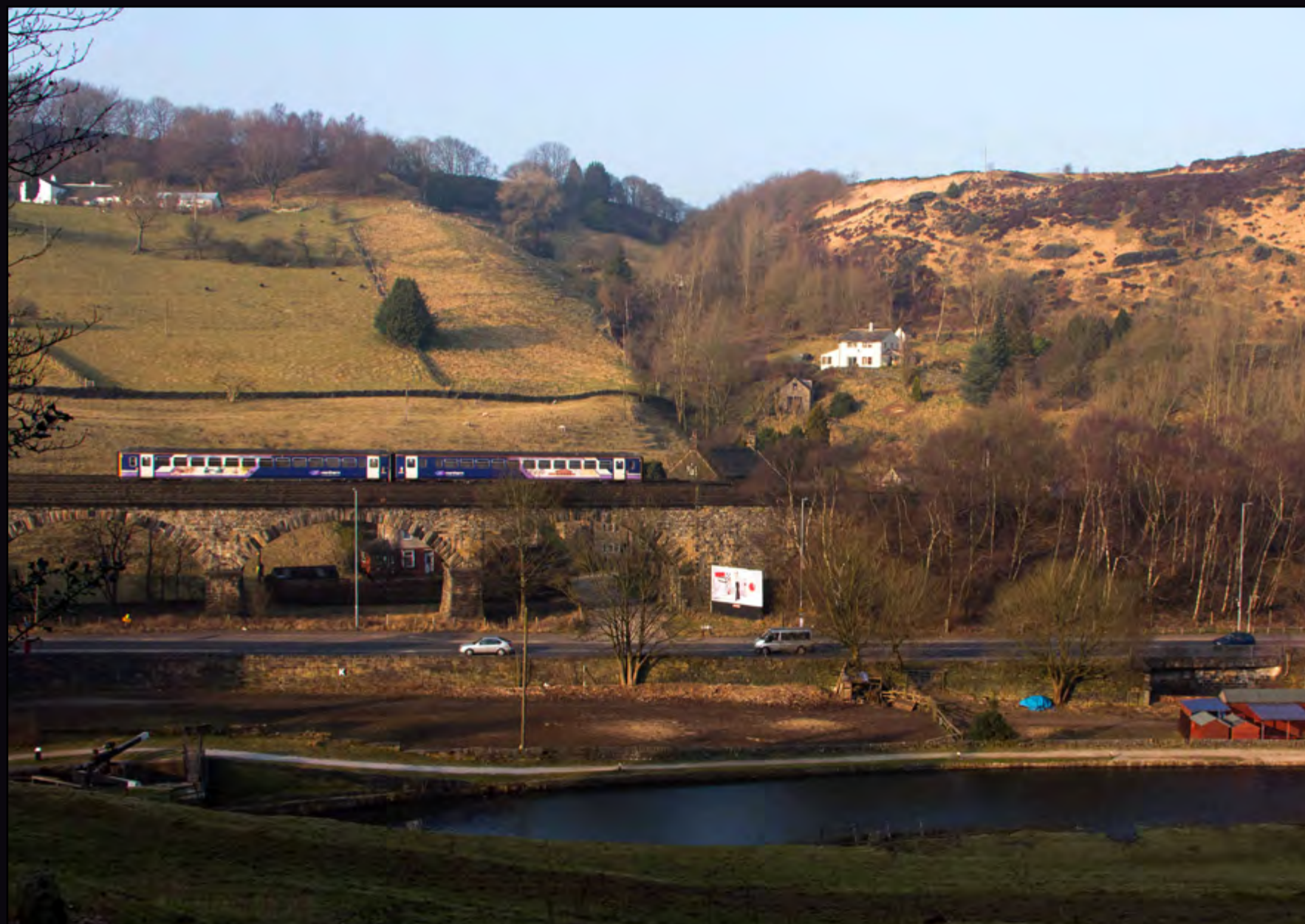
A Northern Rail Class 155 crosses Horsfall Viaduct with a Leeds to Manchester Victoria service on March 15th. Colin Irwin
