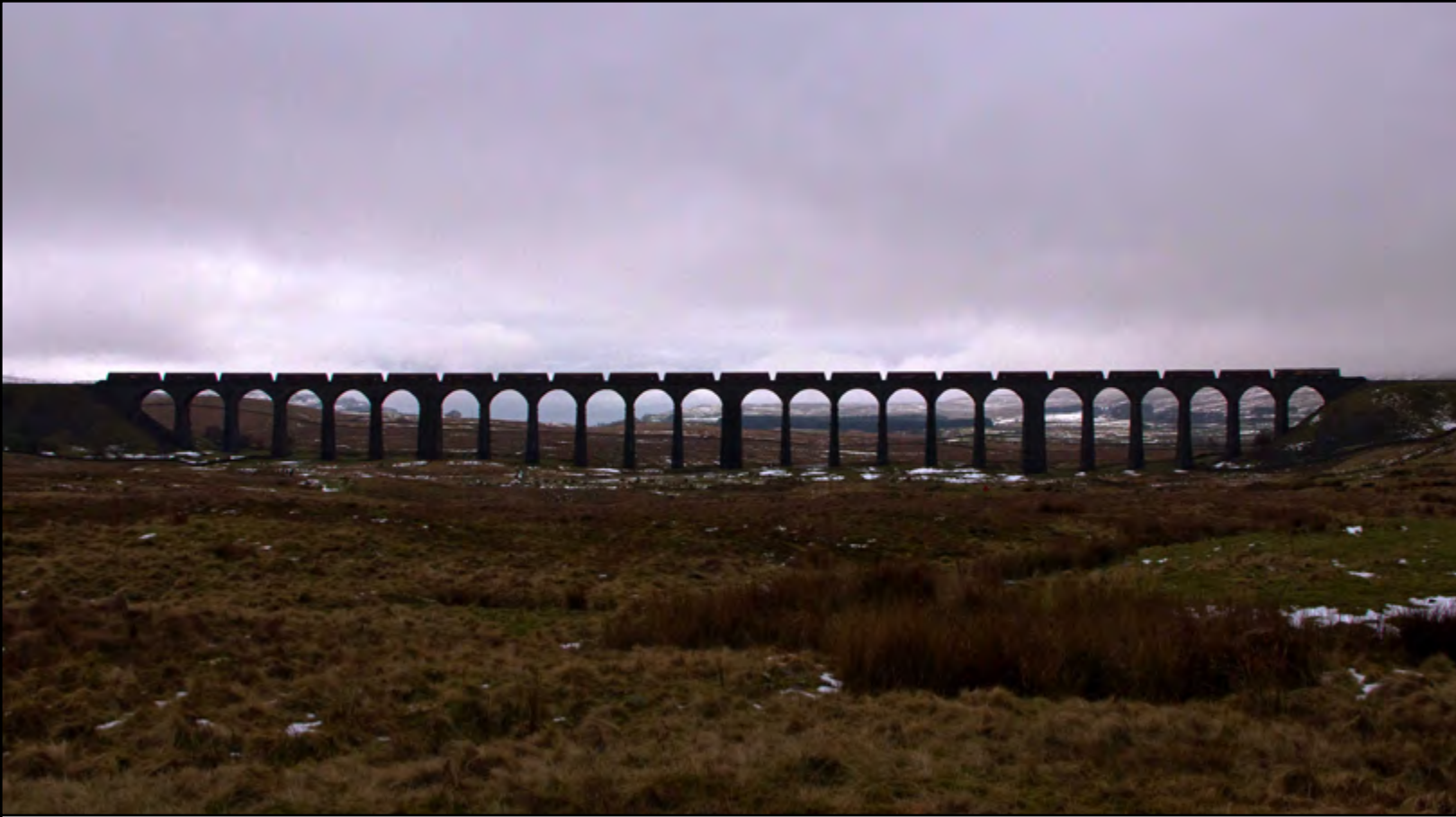
Above: A Class 66 returns north with an empty MGR working, seen crossing Ribblehead viaduct on February 9th. Colin Irwin
